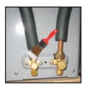
7) Check with leakage detector or soap water if there is any leakage, if not, then put back the copper nuts onto the valves.
