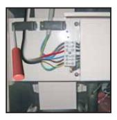
3) Fix the power cable by the wire clip, and then install the front panel back.
