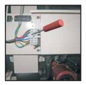
2) Connect the power cable to the terminals on the indoor unit. (Please match the wire colors to the marks on the terminals of both indoor and outdoor units.
