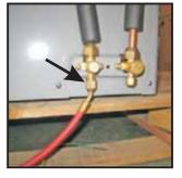
4) Connect the other tube of the pressure gauge to the outdoor unit.
