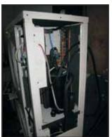
2) Pass the power cable from the indoor unit through the cable gland on the backside of the outdoor unit, and connect it to the terminals of the outdoor unit.
