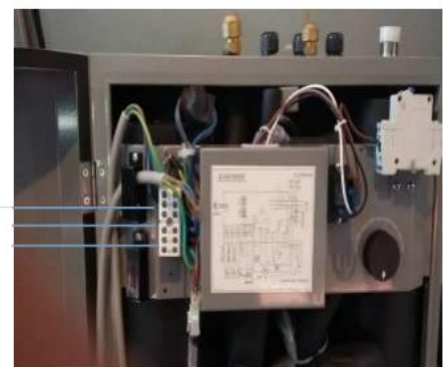
L, N, S must be connected correspondently.
